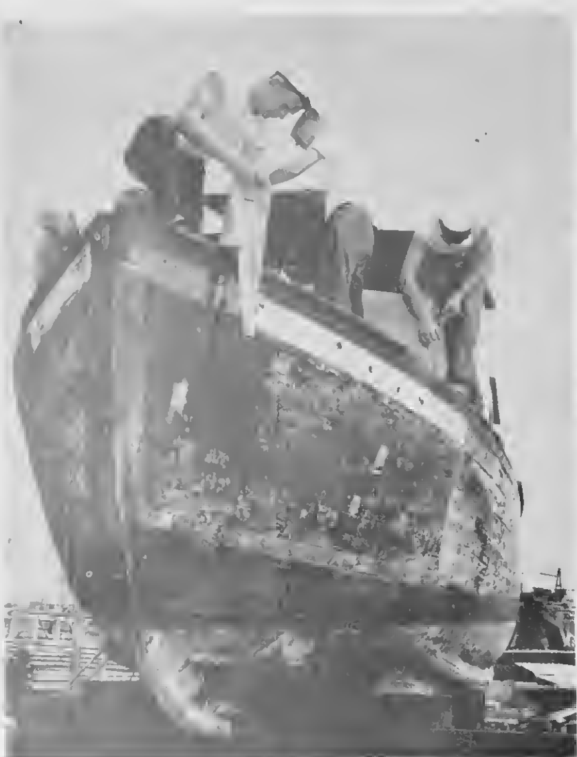
FOR ALL its age and heavy duty, the new Pedernales has trim lines. Doing carpentry work on the cabin are Scouts Artie Spitzer, Phil Heffelfinger and Bruce Clark.
